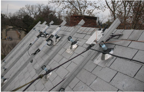
Rails mount on the roof and solar panels mount on the rails
